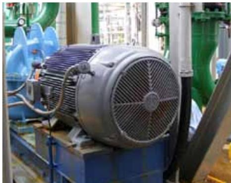
For larger motors rated above 600V, the current is usually measured by a clamp-on power frequency CT, on the secondary of the CT, that measures the supply current to the motor for protection purposes (usually at the MCC). MCSA provides on-line monitoring and analysis of current to assess the condition of an induction motor drive system.
